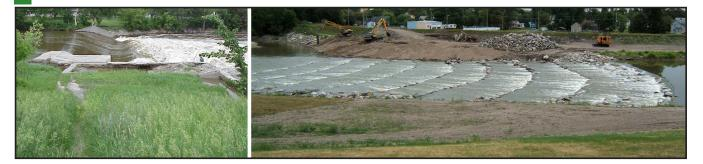
In 2005, a project involving a number of state and local watershed partners removed an old dam in Crookston (left) and replaced it with a series of rapids formed from boulders (pictured from opposite side of river). This project, along with a similar project upstream of town, restored fish passage from the Red River in East Grand Forks to Thief River Falls, a distance of 125 river miles. Fish now have access to better spawning habitat.
